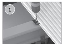
Position the clip with the stop and predrill with a 3 mm bit.
