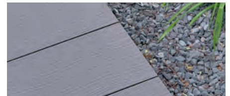
After cleaning with water
